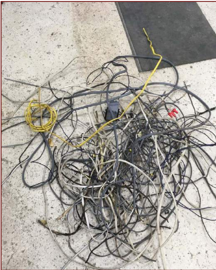
More wires that we removed.
