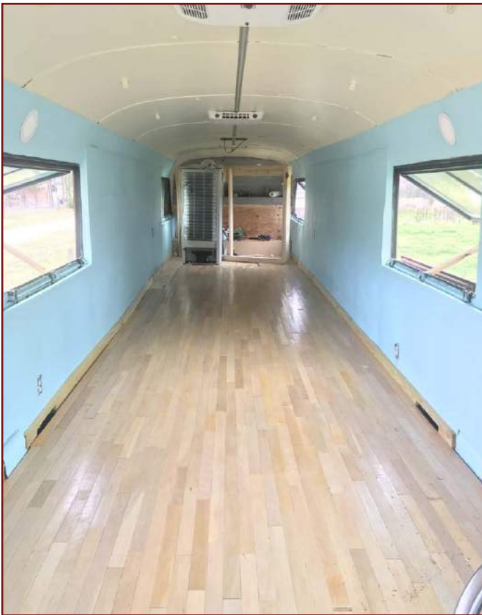
Re-claimed oak flooring is laid.
