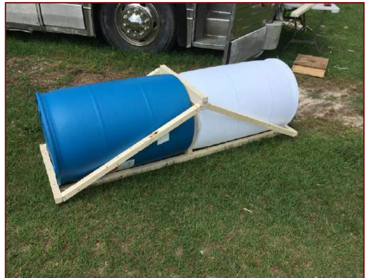
Building a frame for the grey and black water tanks.
