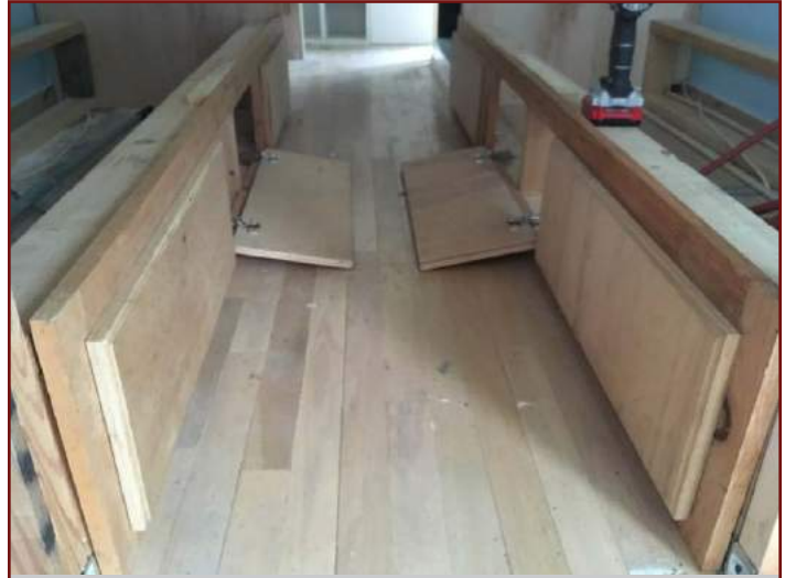
Building the bunk beds with storage underneath.
